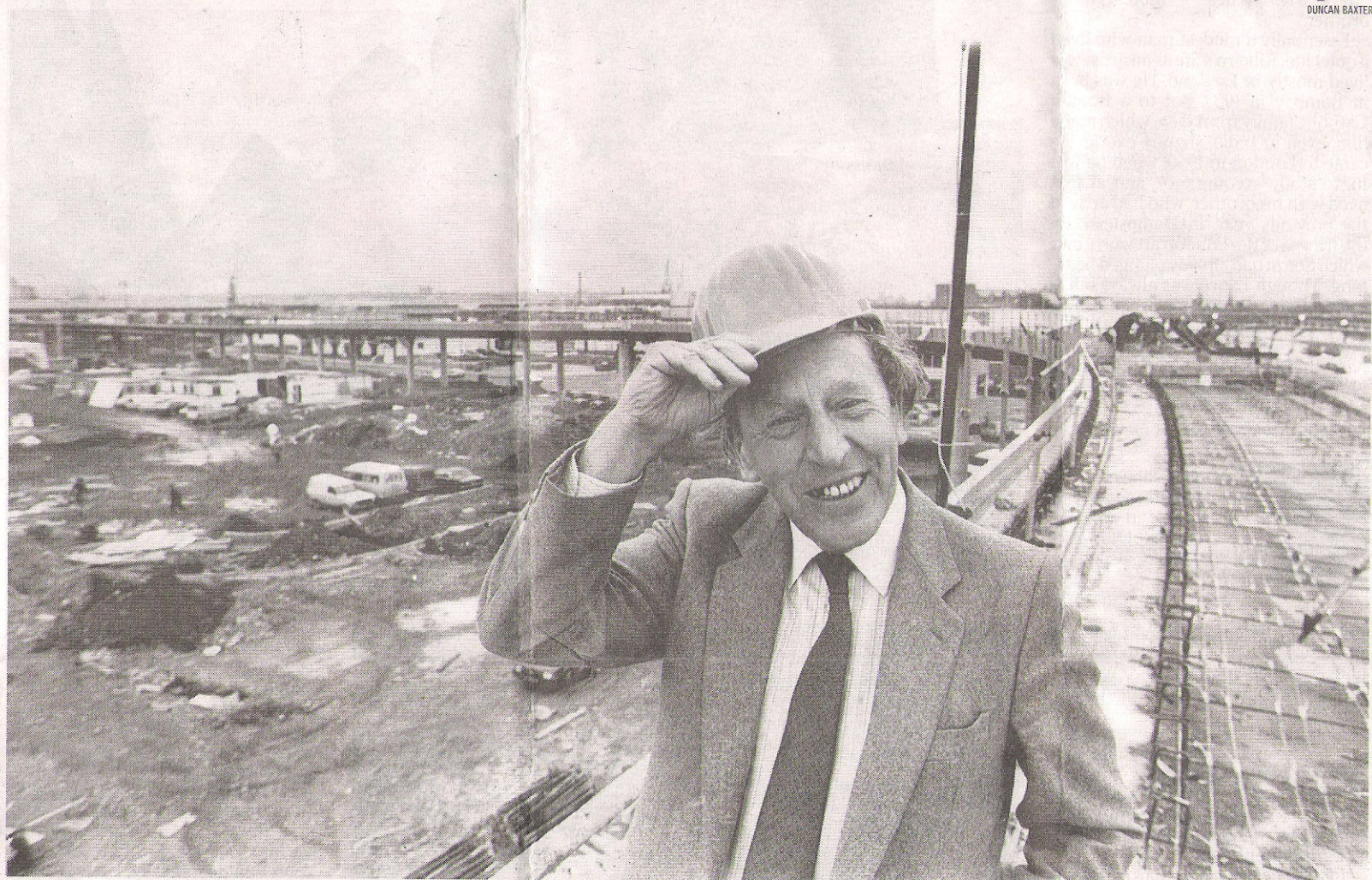
Ward inspects the construction of the DLR in January 1986; and below, the Canary Wharf development on the Isle of Dogs begins to take shape in April 1989
