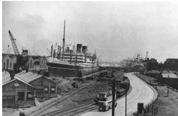
King George V Dry Dock 1984 乔治王五世干船坞
