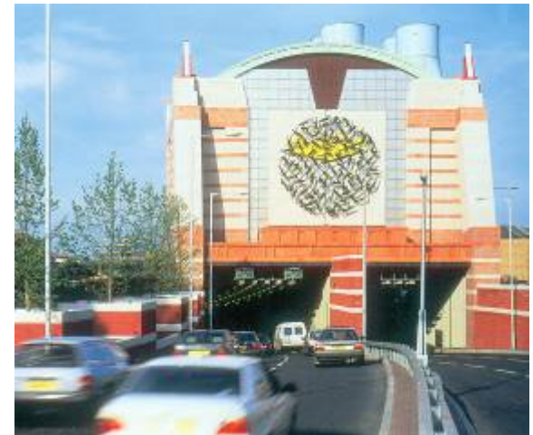
Limehouse Link Tunnel
