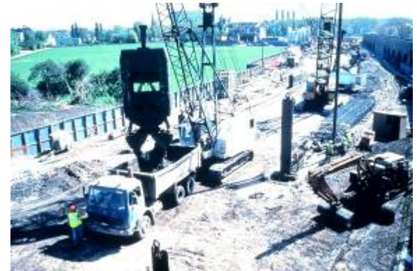
Building the DLR
